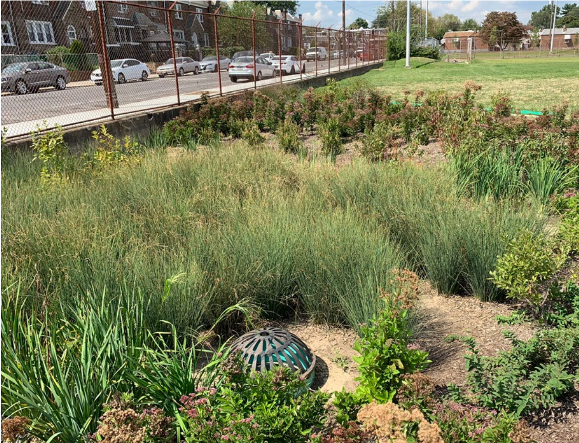
A raingarden installed as part of Philadelphia's Green Stormwater Infrastructure (GSI) projects. GSI are intended to reduce combined sewer overflows, which will ultimately improve the health of the Delaware River.
