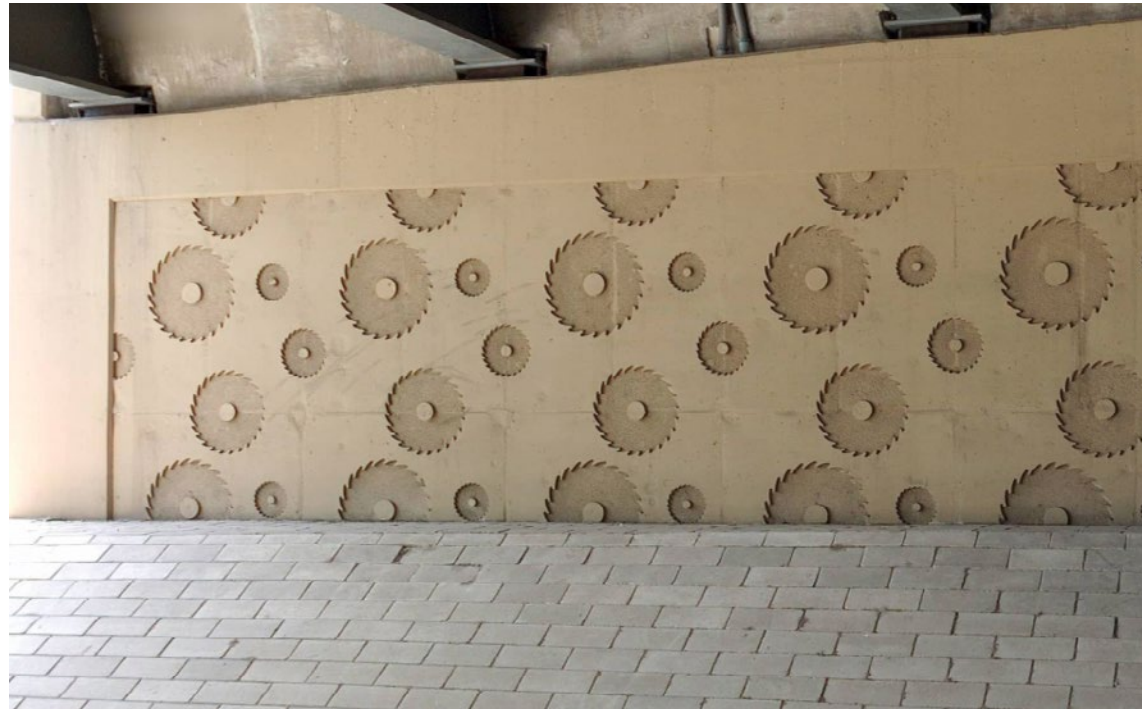
The recently completed Section CP2 of the I-95 reconstruction features this concrete formliner pattern at Unruh Street that celebrates the former Disston Saw Works, previously located nearby.
